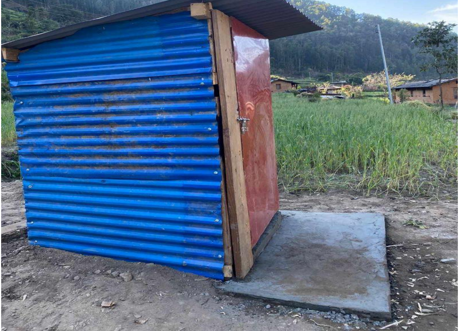
Toilet made of corrugated galvanized iron sheet
